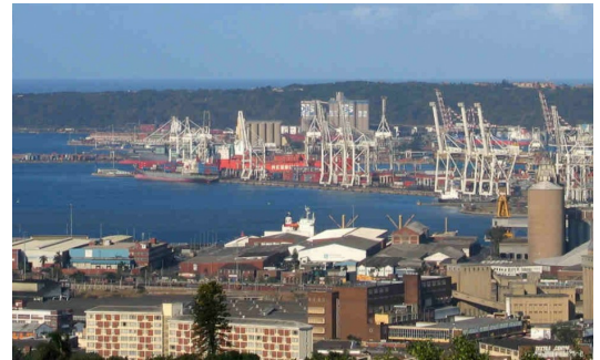
Flooding has hit the Port of Durban Credit: PhillipN
